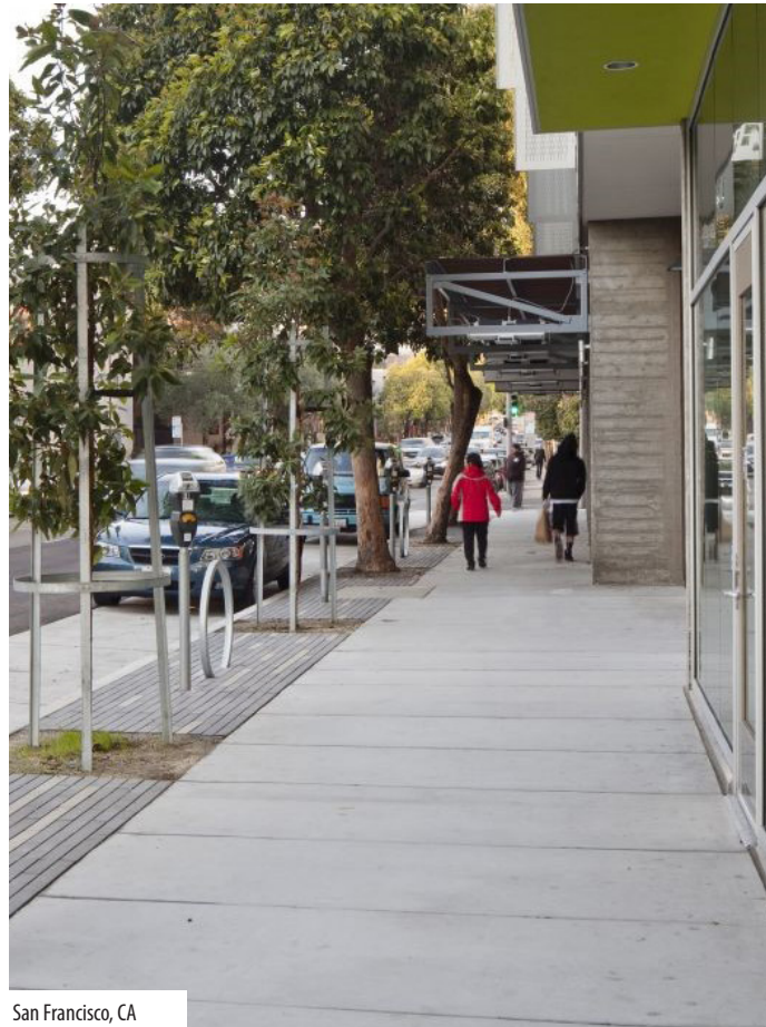
RIGHT Concrete sidewalk with expansion joints spaced 4-feet apart as recommended for streetscape areas in Baileys Crossroads and Seven Corners Image Credit: Andrea Cochran Landscape Architecture
