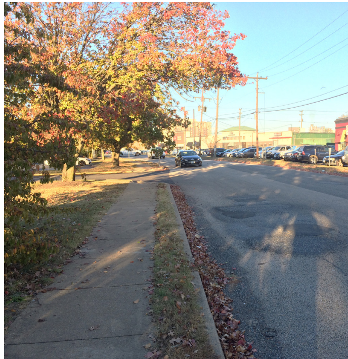
RIGHT Existing conditions for Gorham Street (Collector) in Baileys Crossroads Image Credit: Fairfax County
