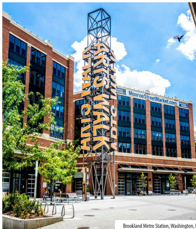
Brookland Metro Station, Washington, DC
