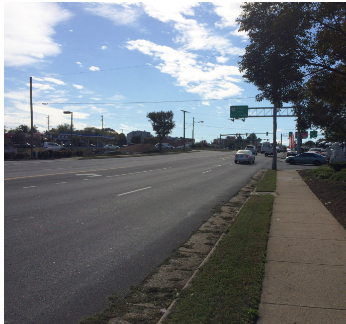
RIGHT Existing conditions for Wilson Boulevard (Avenue) in Seven Corners Image Credit: Fairfax County
