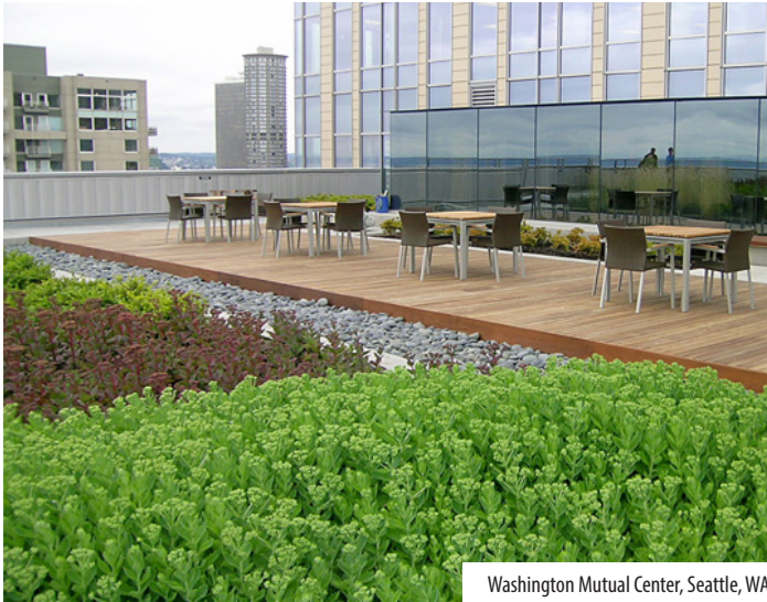
BOTTOM Green roof that combines stormwater capture, native plantings, and outdoor cafe seating Image Credit: ASLA
